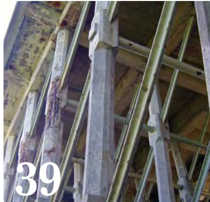
Strengthening Holt Fleet Bridge
