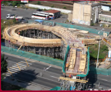
Bílina pedestrian bridge, Czech Republic 38
